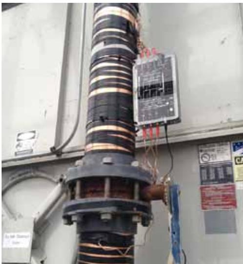
Vulcan S100 installed on cooling towers
