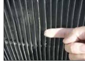
Silica is not removed by hosing, but can be peeled off with a nail.
